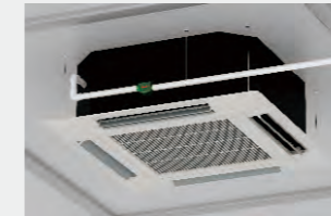
Installed in drainage pipe
